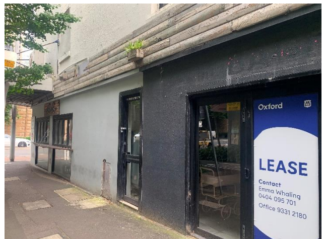
Figure 10 – View of ground floor retail facades on Reservoir Street.
